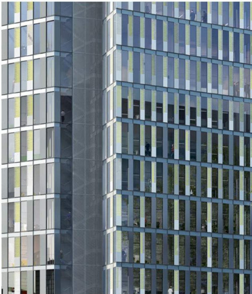
North East Facade
